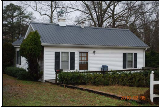
Figure 10: 2010 Photograph of the c.1940 Tenant House
